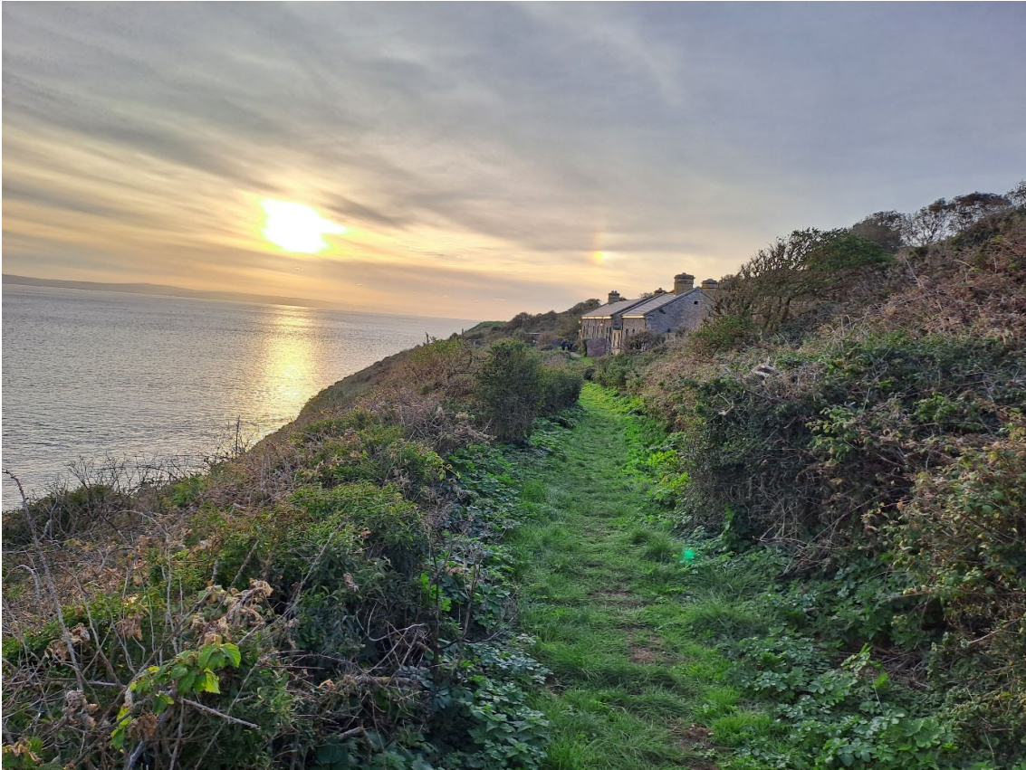
Figure 17: South footpath facing west towards the Barracks buildings.
